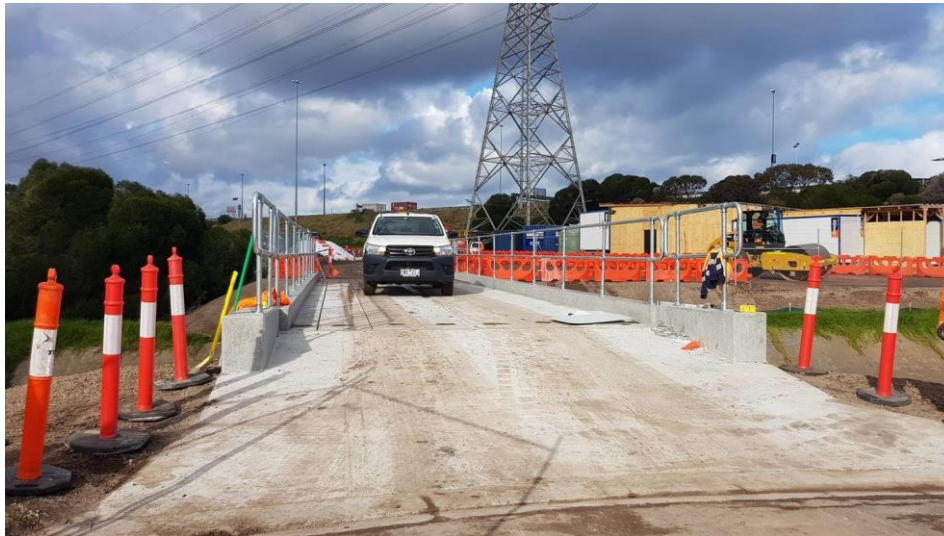
Newly constructed Thomas Street bridge
