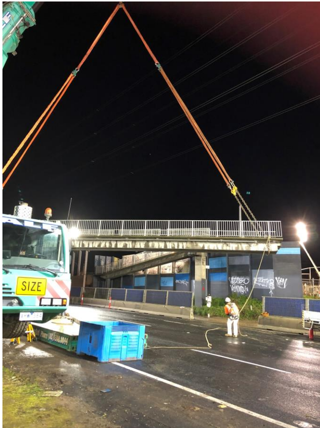
Muir Street pedestrian overpass inbound section
