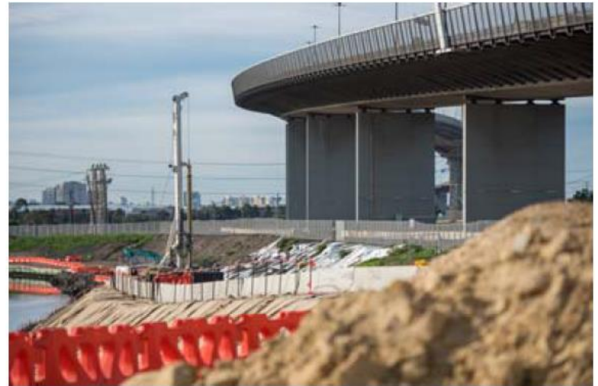
Stony Creek piling
