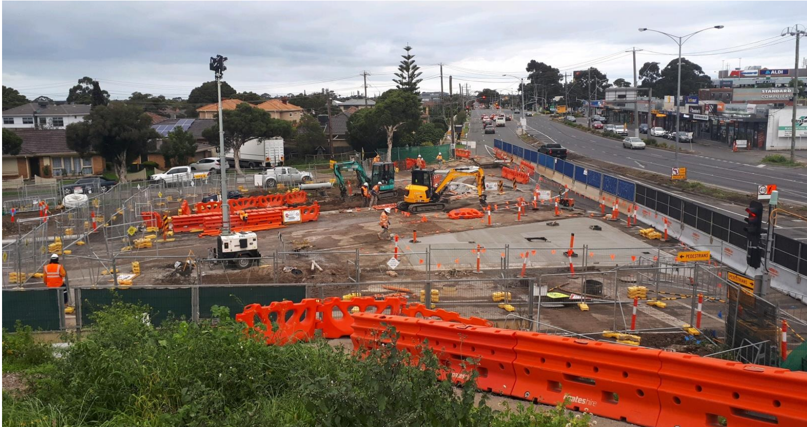
Closure of Millers Road outbound exit ramp and Beevers Street
