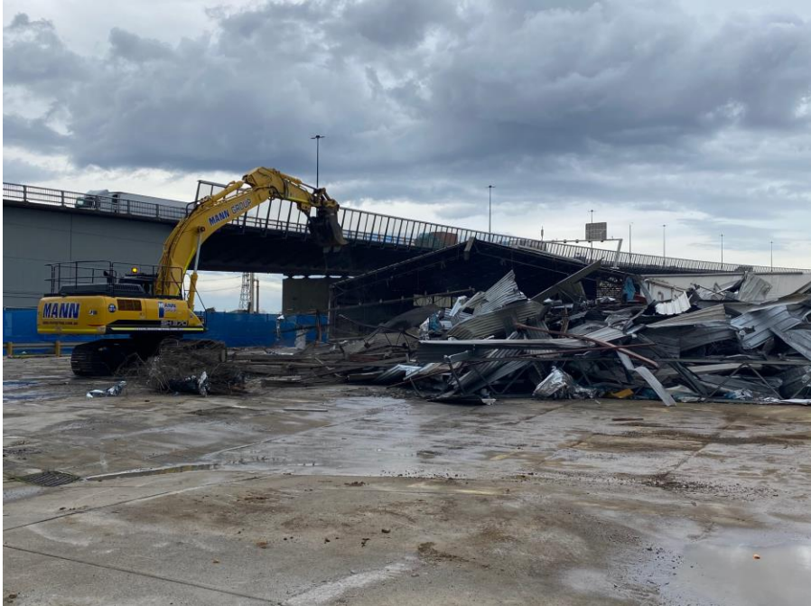
Demolition works at the Socobell site
