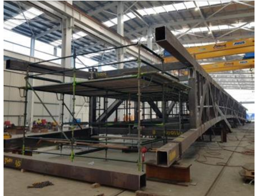
Fabrication is underway for the new walking and cycling overpasses
