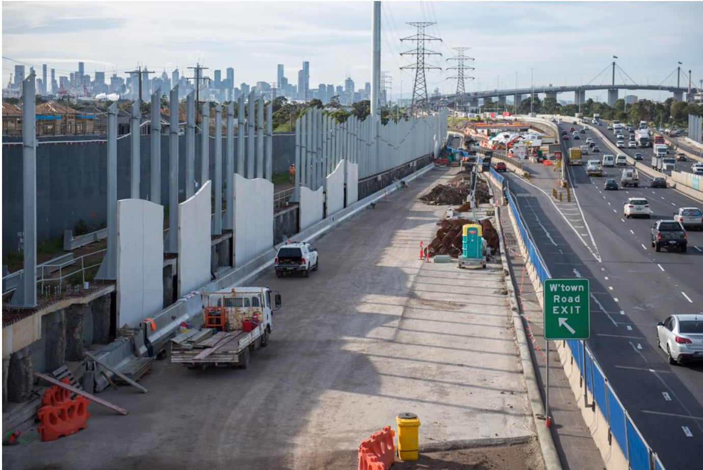
West Gate Freeway widening works – inbound towards Williamstown Road exit
