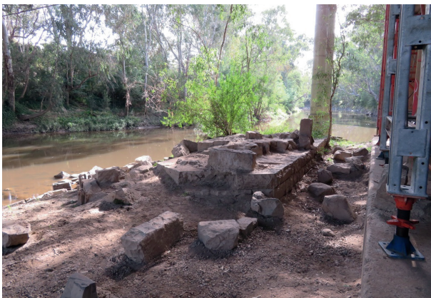
Figure 19-8 Bluestone masonry of Banksia Street Bridges
