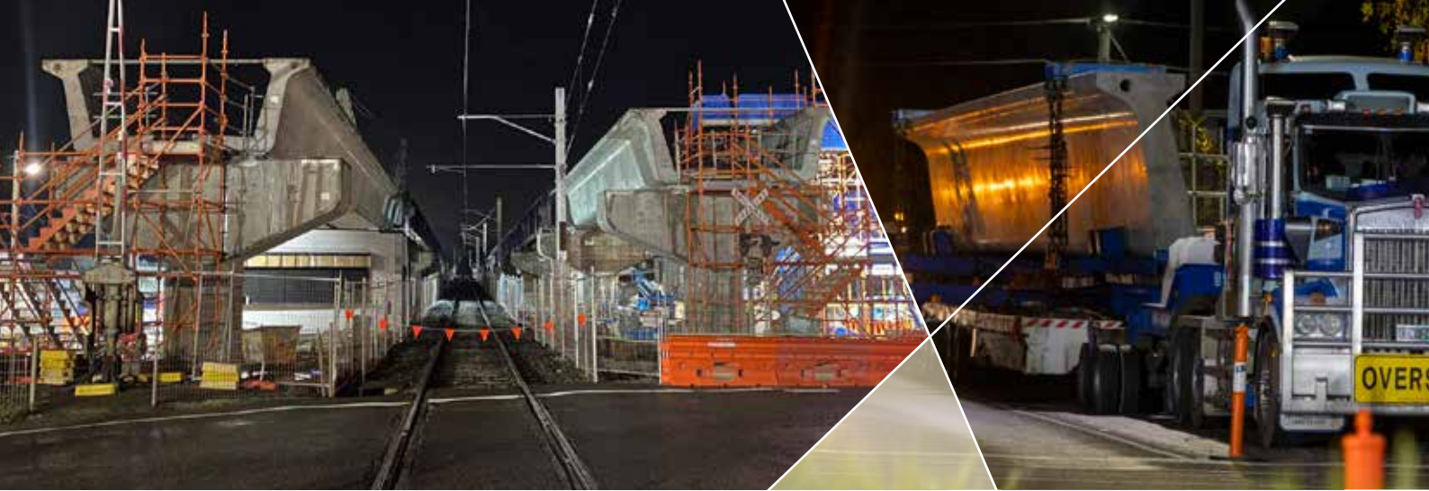
The new bridge viaducts taking shape at Lilydale
