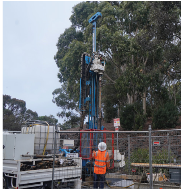
SRL East site investigations at Monash University
