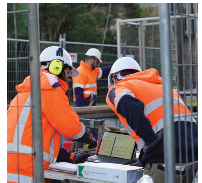
SRL East site investigations at Glen Waverley
