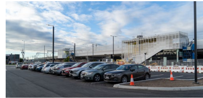
Upgraded north-west car park
